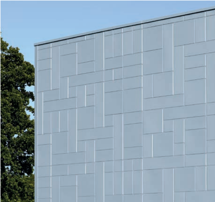
Facade design with random structure, elements from 250 mm to 1000 mm
